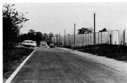
Fig. 6. Typical housing areas, with 'Fishbowl' lanterns surmounting 5m. square GRP columns (above) and steel columns (below)
